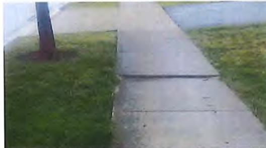
Example of sidewalk trip hazard
