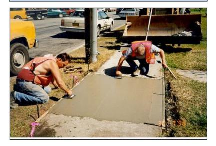
**Replacement:** This is the most common form of repair and is necessary to replace cracked, deteriorated or uneven areas of sidewalk. Sections are removed, reformed, poured, and finished by experienced contractors.
